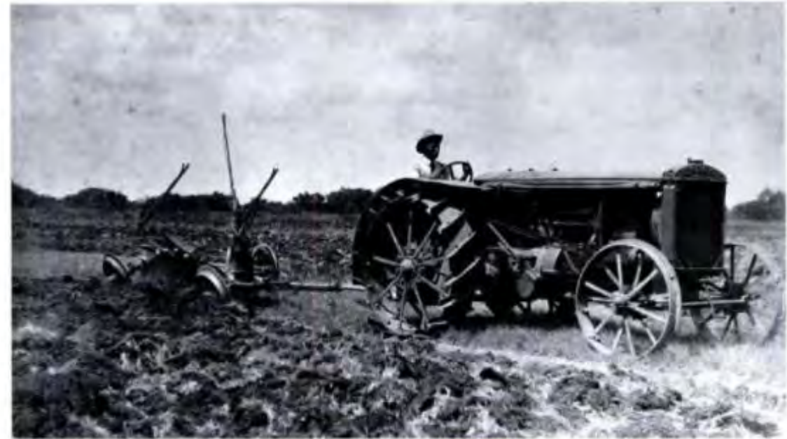
Sam Evers, aboard his Alice Chalmers tractor, levels the air strip at Kelly Field Number 2. In 1917, Evers was paid $25 a day for each of the five tractors he used in the construction.
